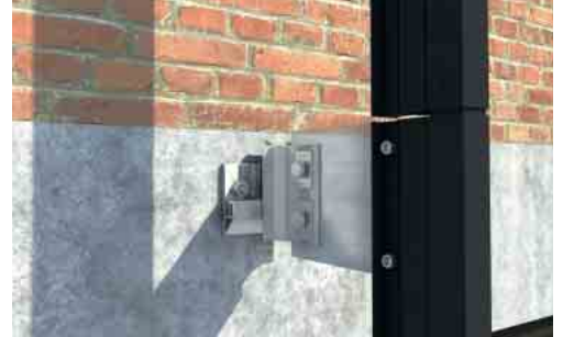
2. Montage der Lisene inklusive Befestigungskonsole am Baukörper 2. mounting plaster strips with fixing bracket to building structure
