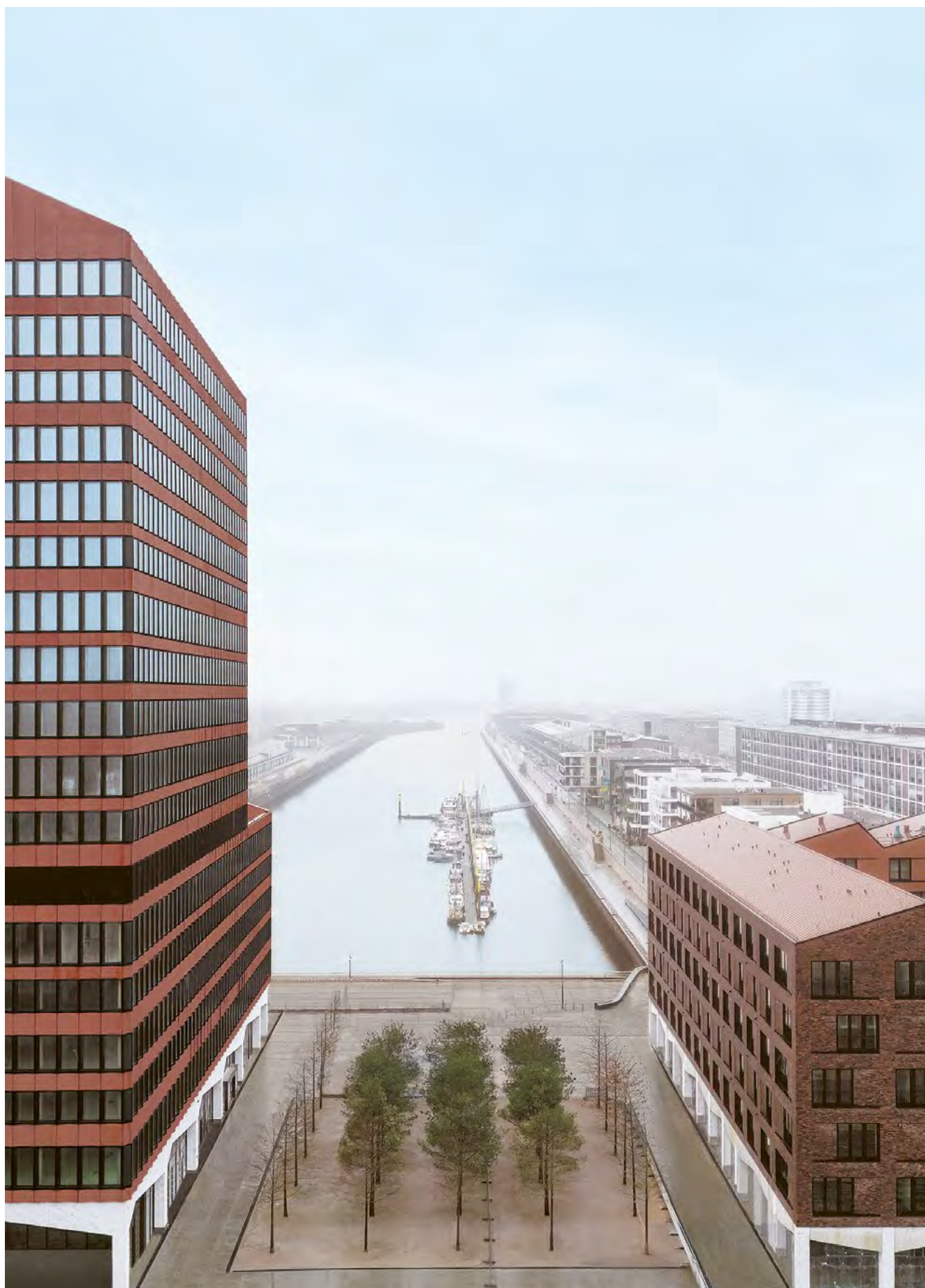
Europahafenkopf Zechhaus, Bremen, Germany © cobearchitects
