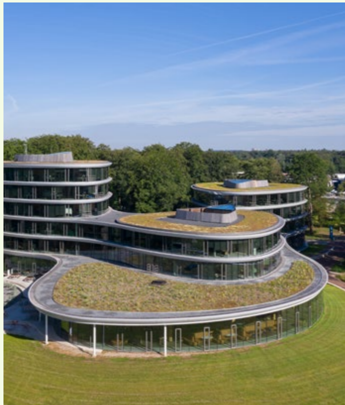
As an energy neutral building that can be completely dismantled, the Triodos Bank office building in The Netherlands with a timber structure and glazed aluminium façade is setting global standards in circular construction.
