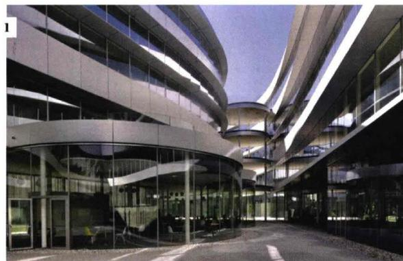
1. UNO DEI CORTILI INTERNI DEL CAMPUS AL PIANO TERRA, SISTEMA PER FACCIATE IN ALLUMINIO **SCHÜCO** FWS 60 CUSTOM CON INSERITI SISTEMI PER PORTE IN ALLUMINIO SCHÜCO ADS 75 HD HI. AI PIANI SUPERIORI, SISTEMA PER FACCIATE IN ALLUMINIO SCHÜCO FWS 60 CUSTOM CON PREDISPOSIZIONI PER AGGANCIO FASCIONI IN LAMIERA. FOTO PHILIPPE RUAULT
