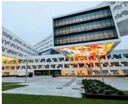
Statoil headquarters, Fornebu, Norway
